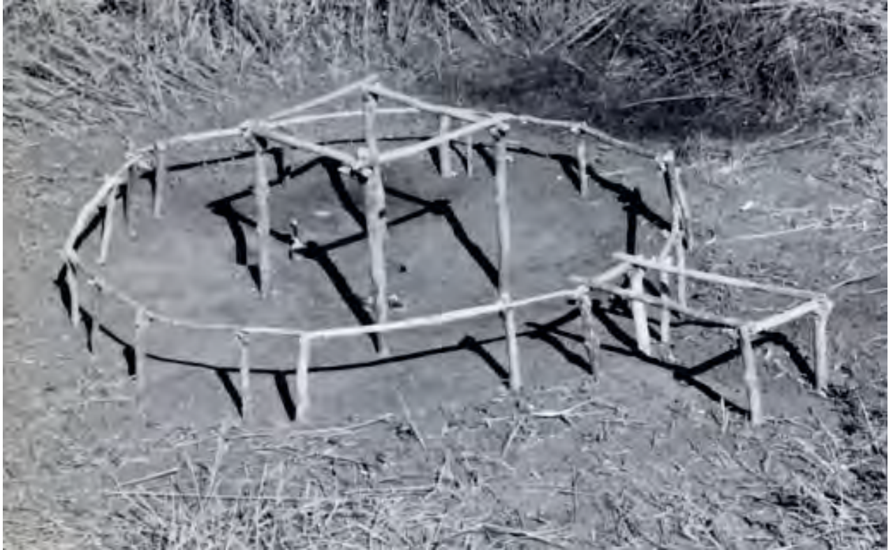
The basic structural framework of the earth lodge is constructed within a shallow pit.
