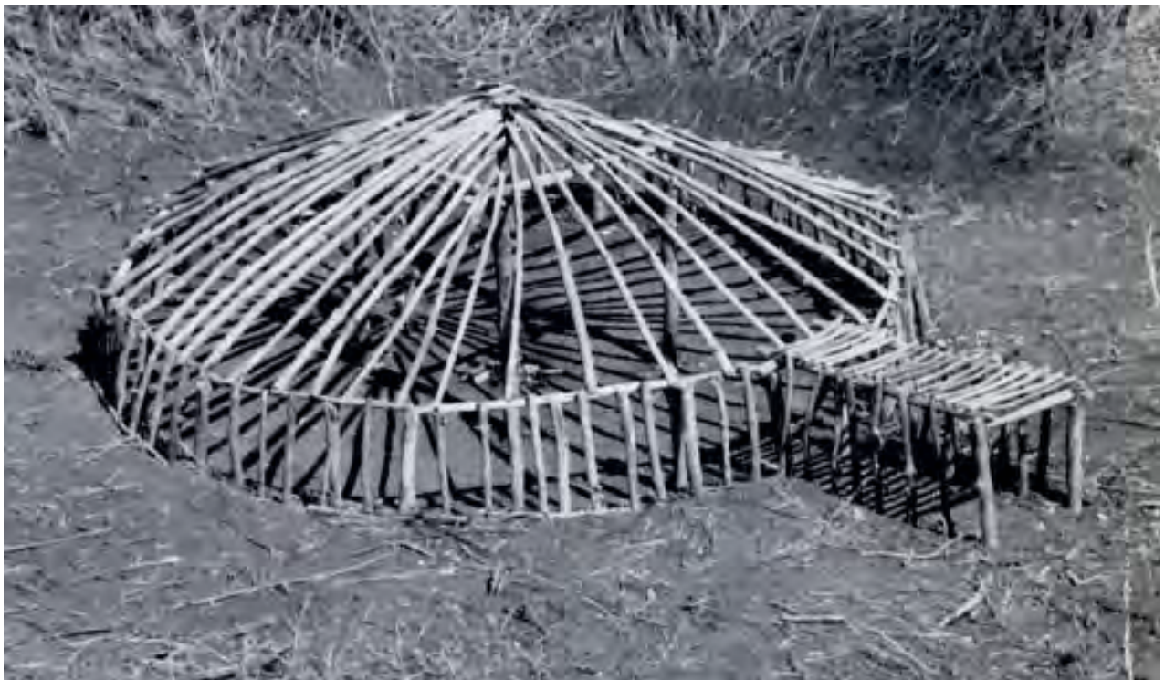
The framework is completed. Next, layers of grass will be added and then a thick layer of earth.
