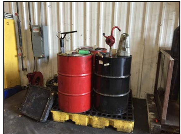
Before: Lubrication storage facility
