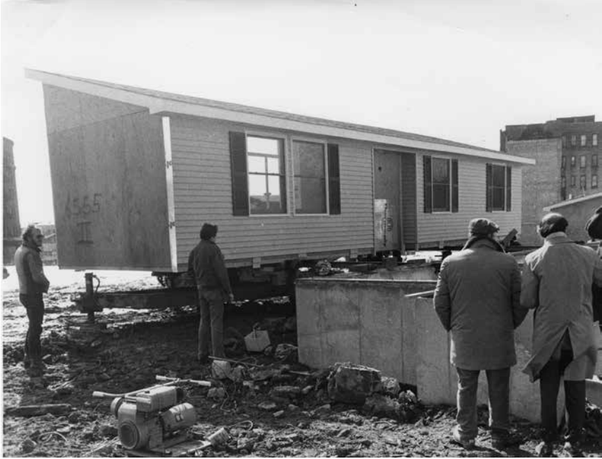
Prefabricated, single-family houses for purchase, with large subsidies, going up in Charlotte Gardens in the South Bronx during the early 1980s. (COURTESY OF PETER BRAY.)
